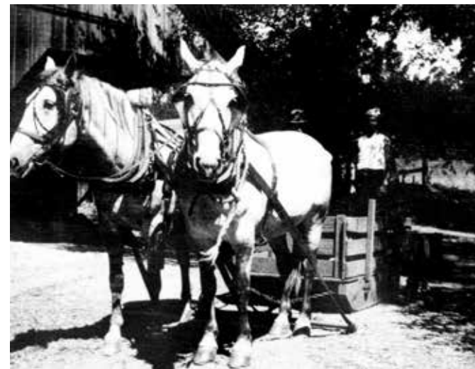
A horse-drawn farm sled at the Rowland Ranch in 1907. Farm sleds were commonly used to transport heavy or bulky agricultural goods across uneven or soft ground where wagons with wheels might sink or become difficult to pull.
